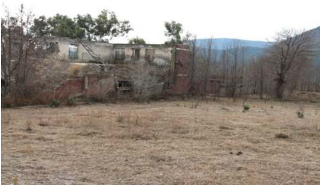
A public school in a rural village in Orakzai
